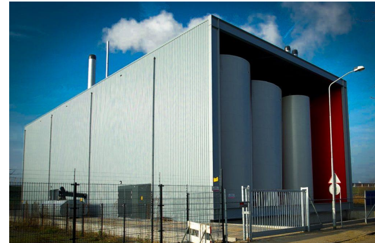
Wood chip fired boiler 5000 kW
