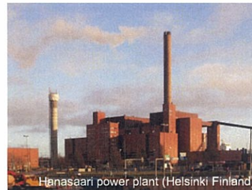
Hanasaari power plant (Helsinki Finland)
